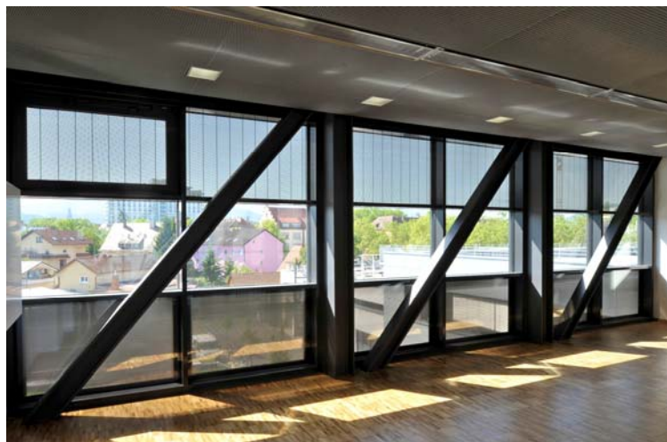
New laboratory building at Fraunhofer ISE: Seminar room with building-integrated photovoltaics (BIPV), partly transparent PV module with angularly selective transmission (PV-Shade®). ©Fraunhofer ISE
